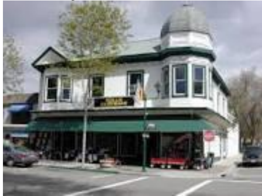
Kolln Hardware Building c. 1890
